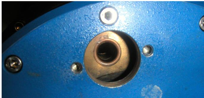
6. Remove the seal bleed hose and compression fitting from the T fitting on the absorber.
